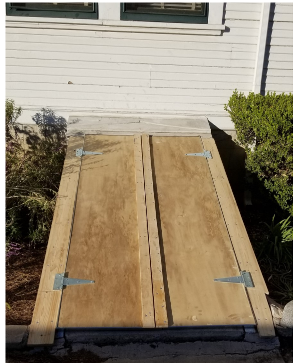
New cellar doors, waiting for fresh, white paint, provide more security.
